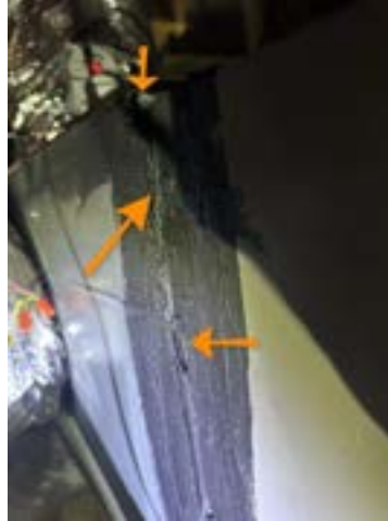
Attic, HVAC unit, openings & condensation
