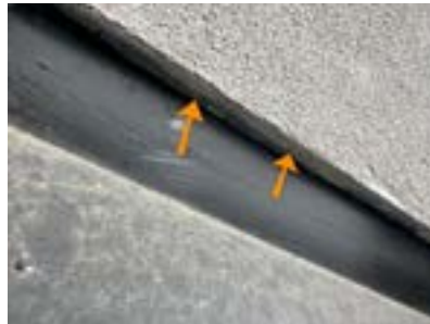
Stucco siding, weep holes, covered
