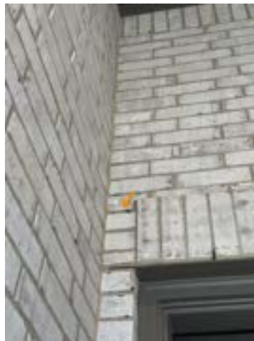
Front of home, brick mortar, gaps Front of home, brick mortar, gaps
