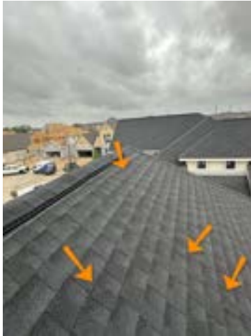
Roof, shingles, excessive scarring
