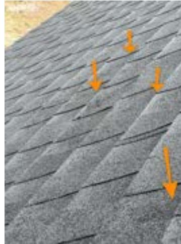
Roof, shingles, excessive scarring
