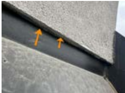
Stucco siding, weep holes, covered
