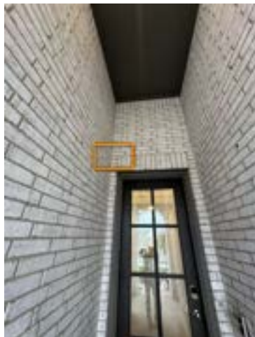
Front of home, brick mortar, gaps Front of home, brick mortar, gaps
