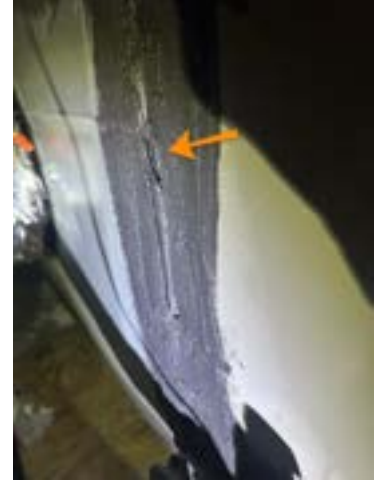
Attic, HVAC unit, openings & condensation
